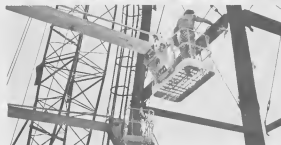
GIRAFFES LIFTED the men with the cutting torches to the designated height at which the legs were to be cut. APARATO DI tipo giraf a hiza e hombernan cu nan torcha di corta na e altura necesario na unda e pianan meser a worde corti.
